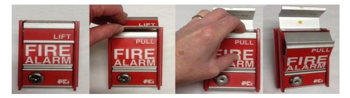
To activate this type of fire alarm pull station, lift up the flap, grasp the top of the device and pull towards you. You will hear a click, and the device will lock into position.
