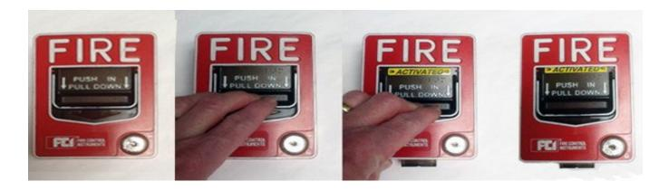
This newer style fire alarm pull station requires that you push in and then pull down. Please note - the "*Activated*" sign will appear when the device has been triggered.
